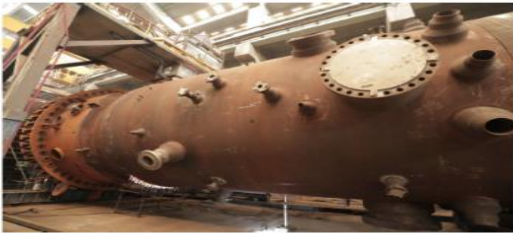
Skirt # SH 1+2+3 - 1 st Gasifier
