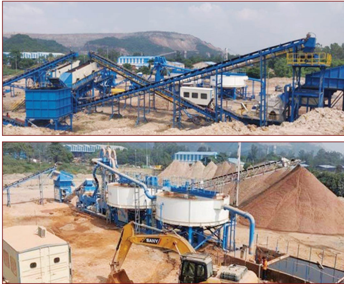
Overburden to M-Sand Plant at Amlohri Plant at NCL
