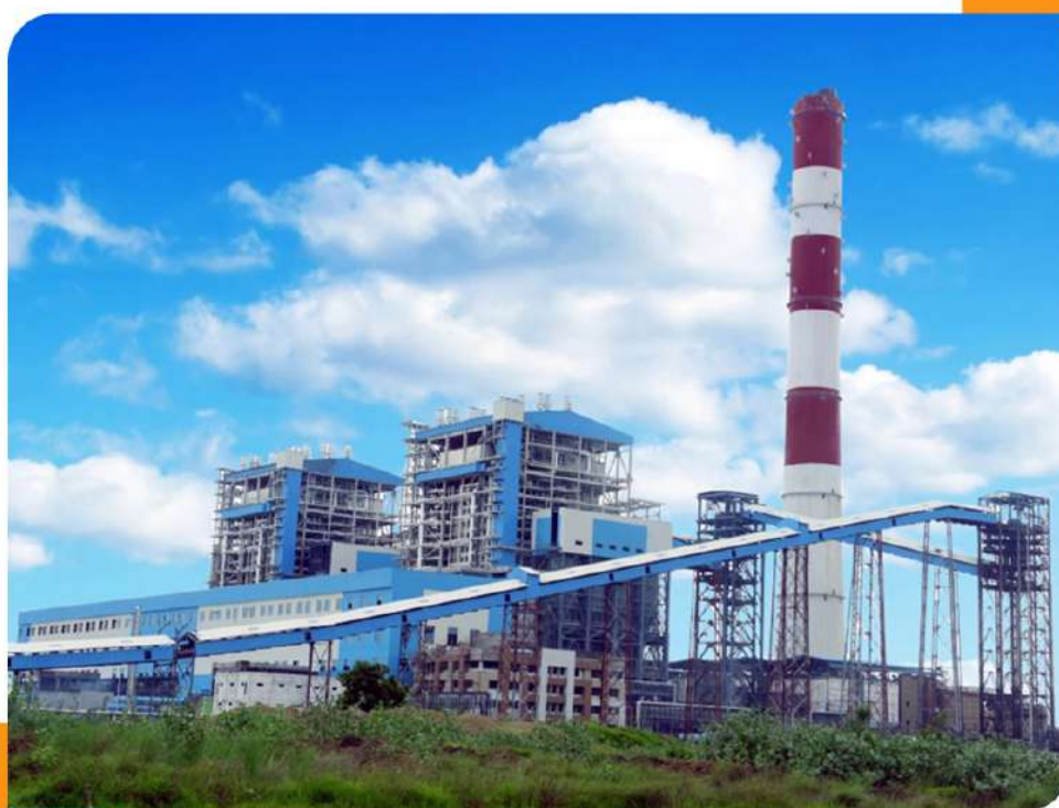
SINGARENI THERMAL POWER PLANT 2X600 MW, SCCL
