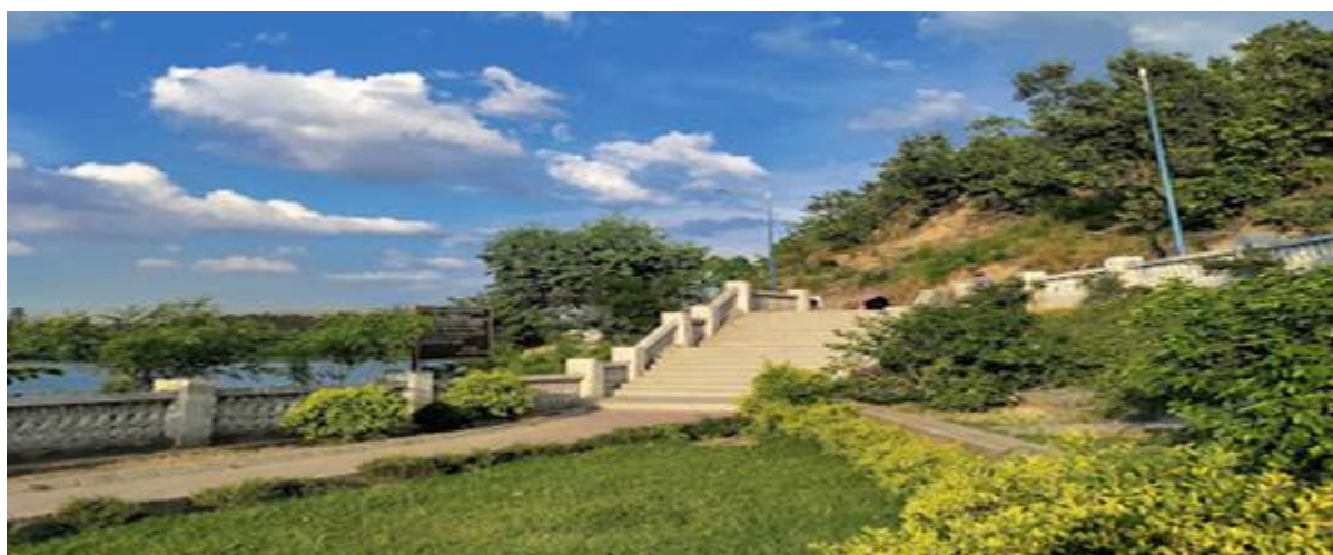
Walkways in Mudwani Dam Eco-Park
