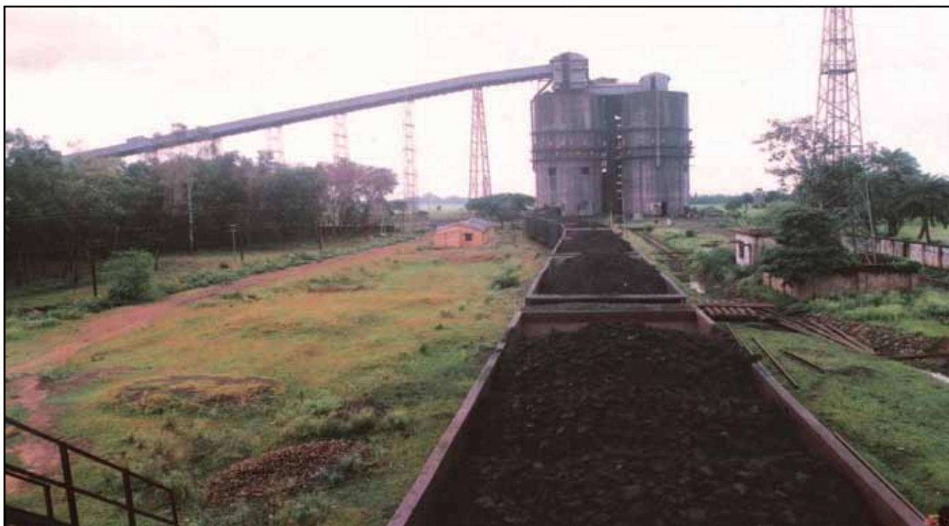
Despatch of Coal to consumer through auto wagon loading system
