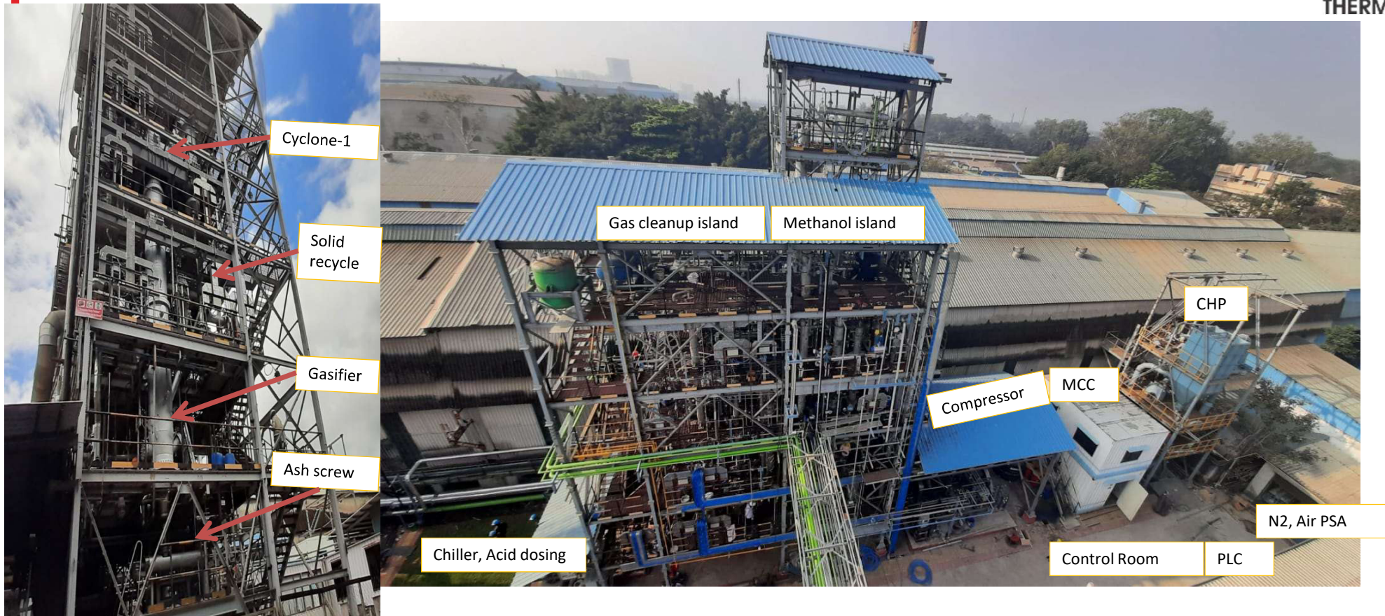
Front view Gas clean up and Methanol plant
