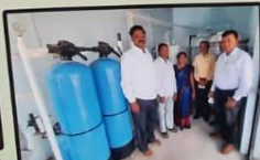
RO plant Piraya village
