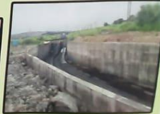
Railway Under Pass (RUP)
